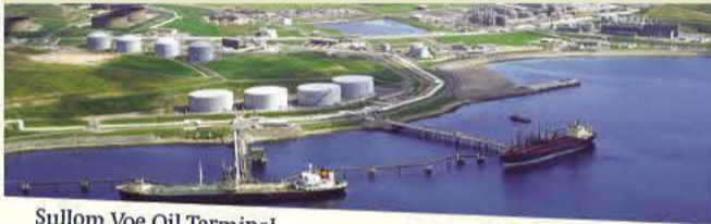
Sullom Voe Oil Terminal
